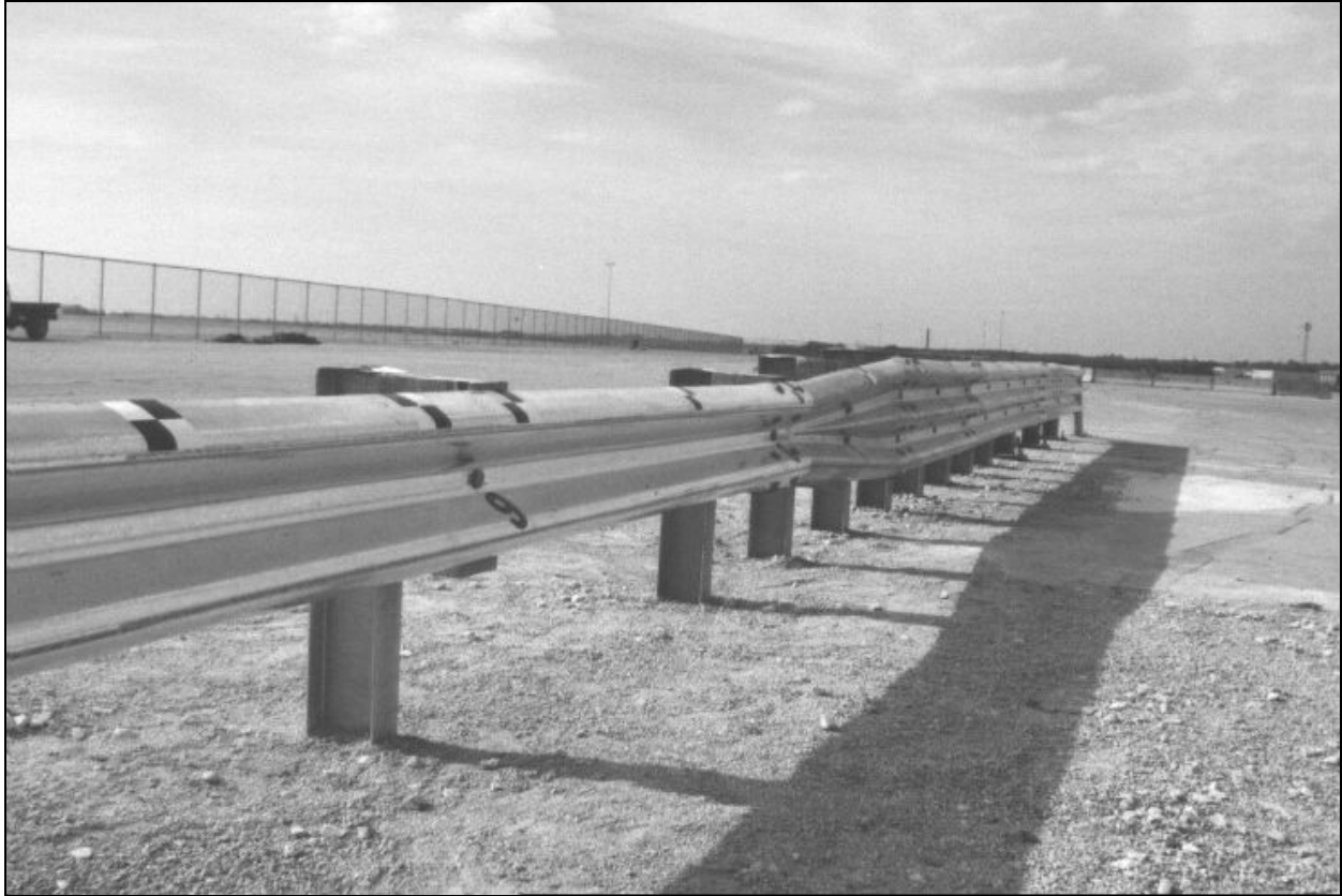
FIGURE 1 Missouri W-Beam to Thrie-Beam Transition (MWT-1 through MWT-3).
